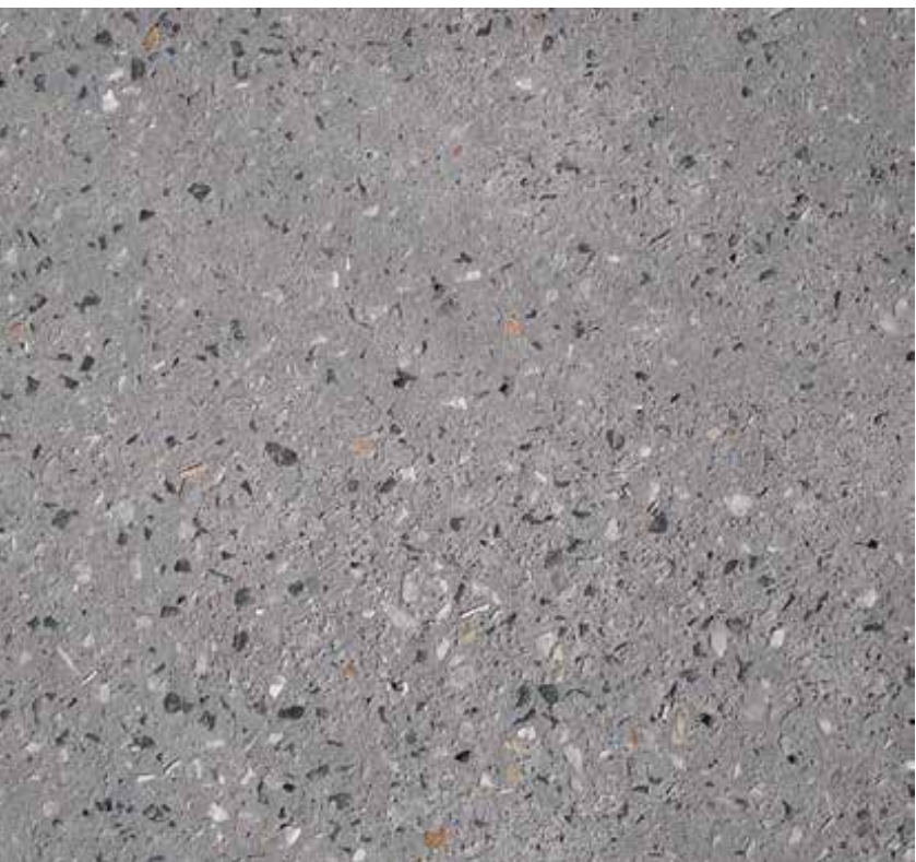
Item Insitu Concrete
